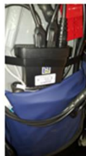
B)Place the light module in the designated location
