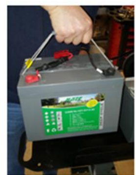
Ready to change the batteries. The procedure is performed in reverse order to insert new batteries
