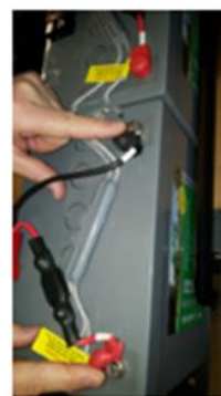
Remove the battery terminals
