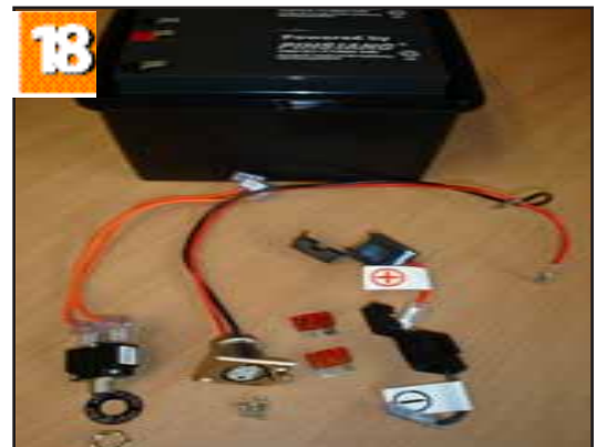
18. Shows the batteries, fuses, power cut out and connection / charger socket.
