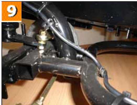
9. Using long-nosed pliers and wire cutters release the tiller cable from its ties.
